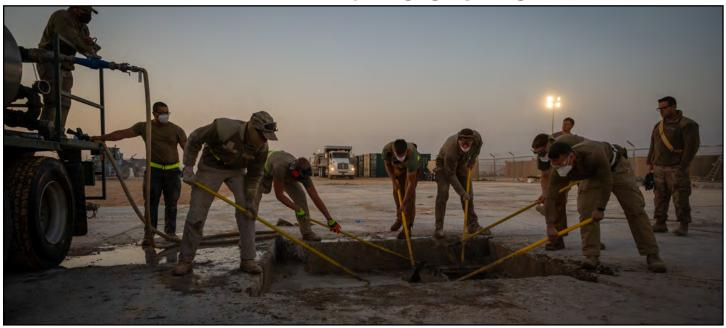
332d Expeditionary Civil Engineer Squadron Airmen mix water and a quick-dry filler to repair runway damage during a rapid airfield damage recovery exercise at an undisclosed location in Southwest Asia, May 12, 2022. RADR exercises test the ability of the 332d ECES to rapidly repair runways and runway support structures to recover and resume airfield operations after it has experienced significant damage. (U.S. Air Force photo by Master Sgt. Christopher Parr)
